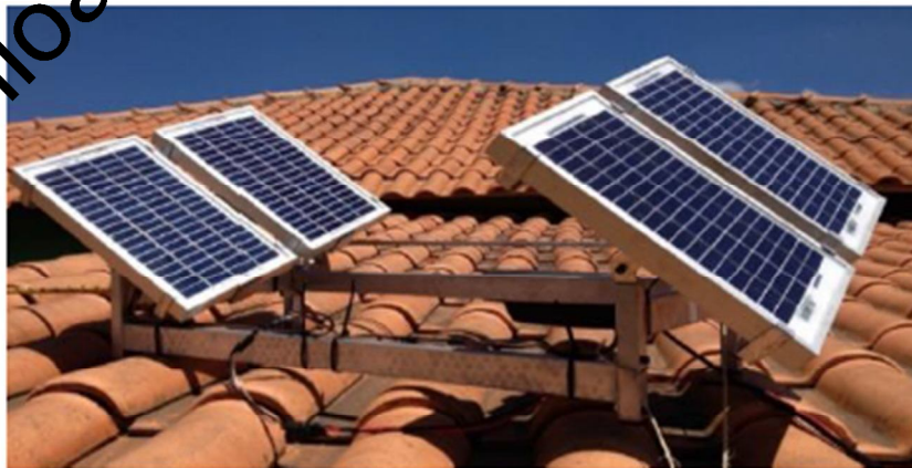
Figure 6. Installation of Sunflower Prototype.
