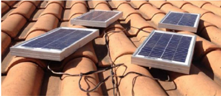
Figure 7. Installation of PV Panels.
