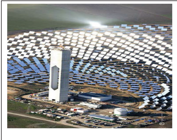
Figure 3. The PS10 solar tower power plant
