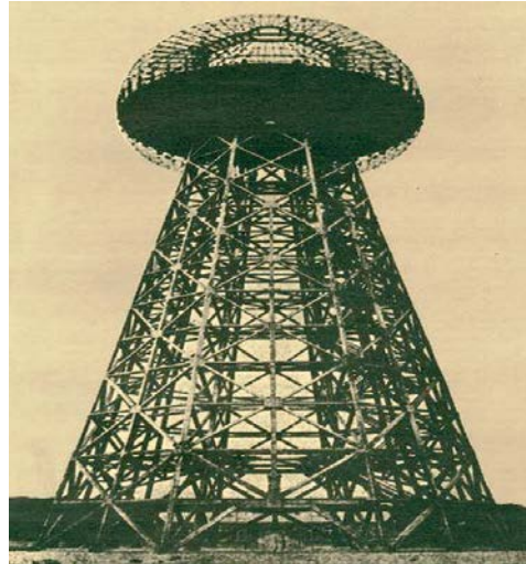
Fig.3. Wardencliff tower located in Shoreham, New York [10]
